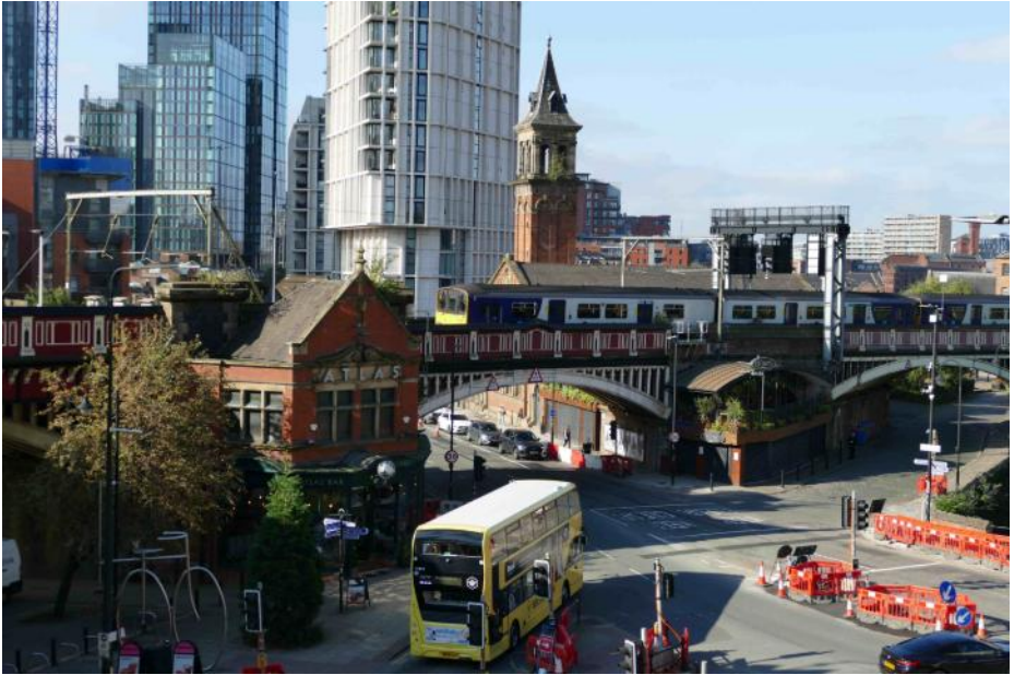
150129 enters Deansgate Station on 18 September 2024 with an ADL E400mmc bus passing below showing the new yellow livery of the Manchester Bee Network franchised buses. Robert Aveyard
