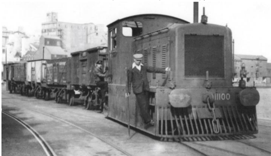
11100 (D2200) complete with full tramway protection working on the dockside at Ipswich in the early 1950s.
