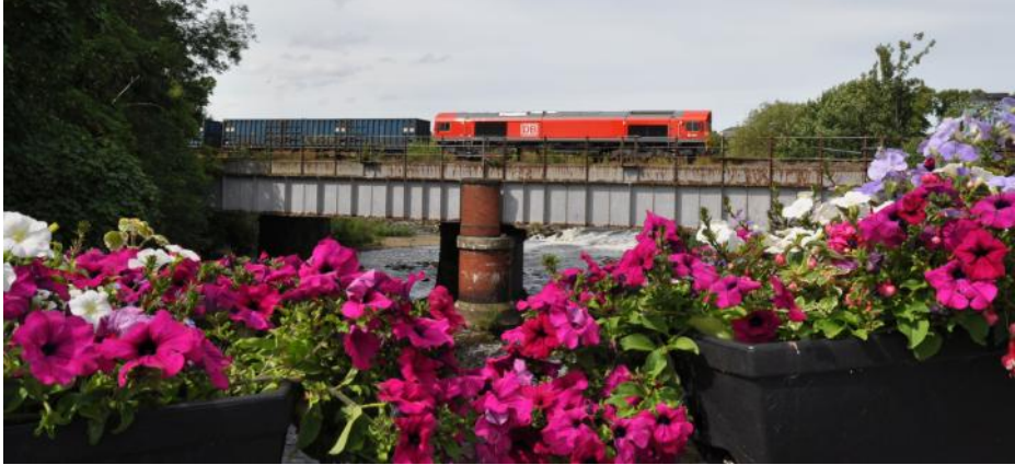
A slightly different view at Newgate Bridge Mirfield.
