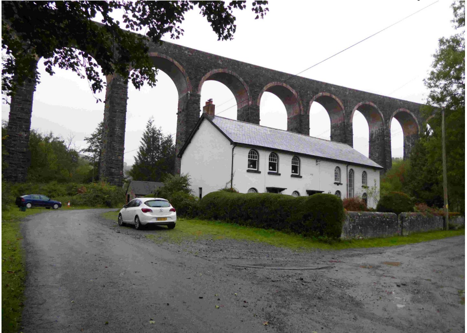
Cynghordy Viaduct 4 October 2022. See article on the Heart of Wales line stations (part 2) by Paul Carpenter from page 4.
