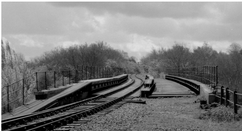
Plate 3. The girder reinforcements, April 1977. Photo: C. Divall.
