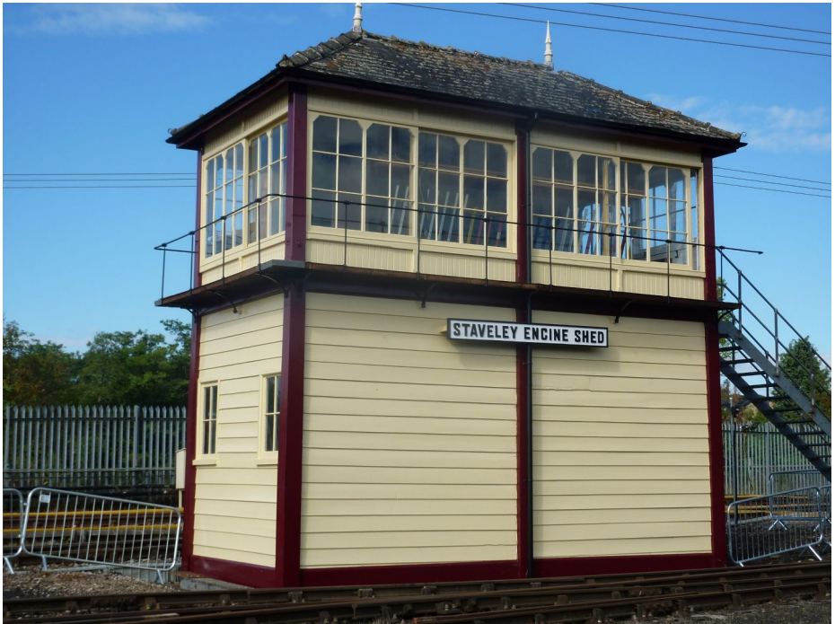
Staveley Engine Shed box at Barrow Hill. See article from page 20.
