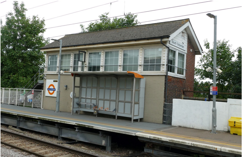
South Tottenham signal box on the Gospel Oak to Barking line seen on 21 July 2022. See article from page 3. Ken Aveyard
