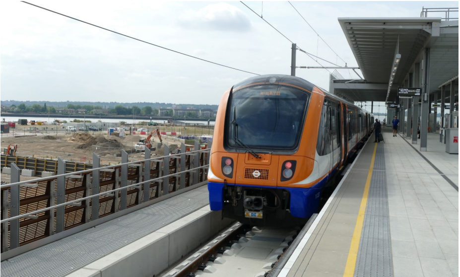
710257 at Barking Riverside on the fourth day of service. The terminus is perched high above the surrounding land which looking towards the river is largely derelict. Looking inland is rather more developed. KA
