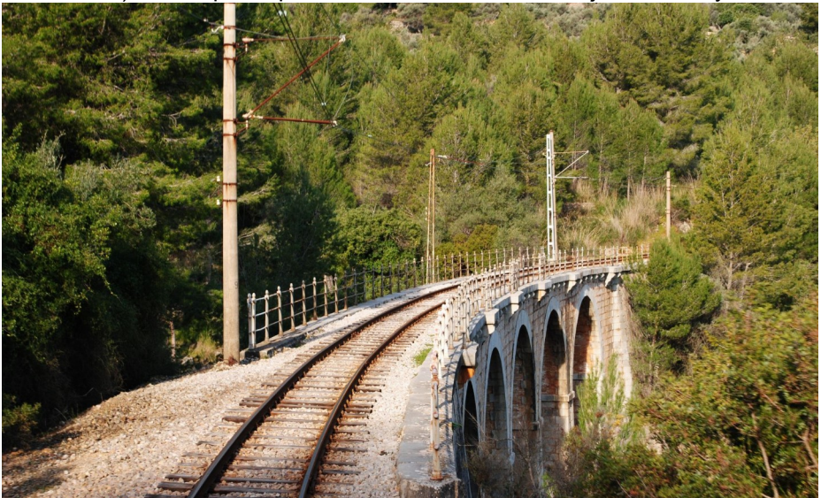
The five arch 'Cinq Ponts' viaduct some 50m high in the Sierra de Alfàbia range.
